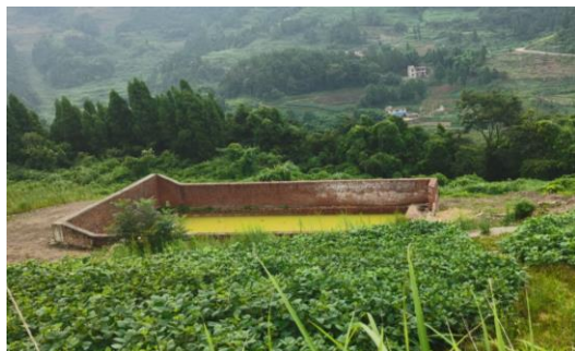
钻井平台放喷坑
