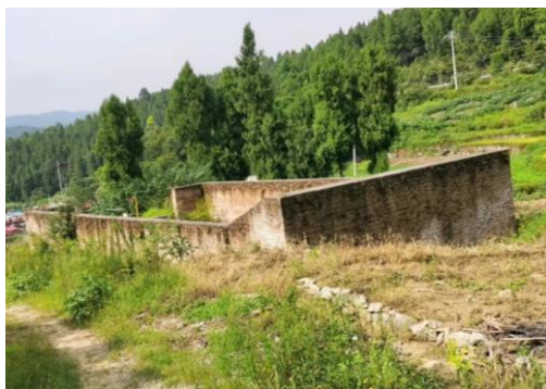
钻井平台放喷坑
